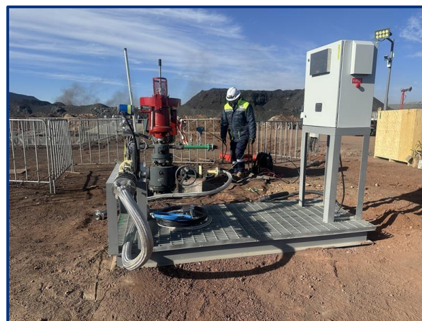
Completion and final commissioning of the additional Lucky Fox pilot wells
