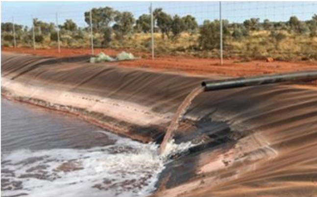
Image: Typical HDPE lined Water Pond
