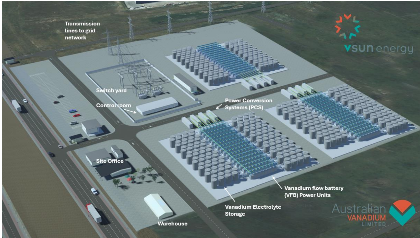
Example 50MW 10-hour (500MWh) VFB BESS Layout
