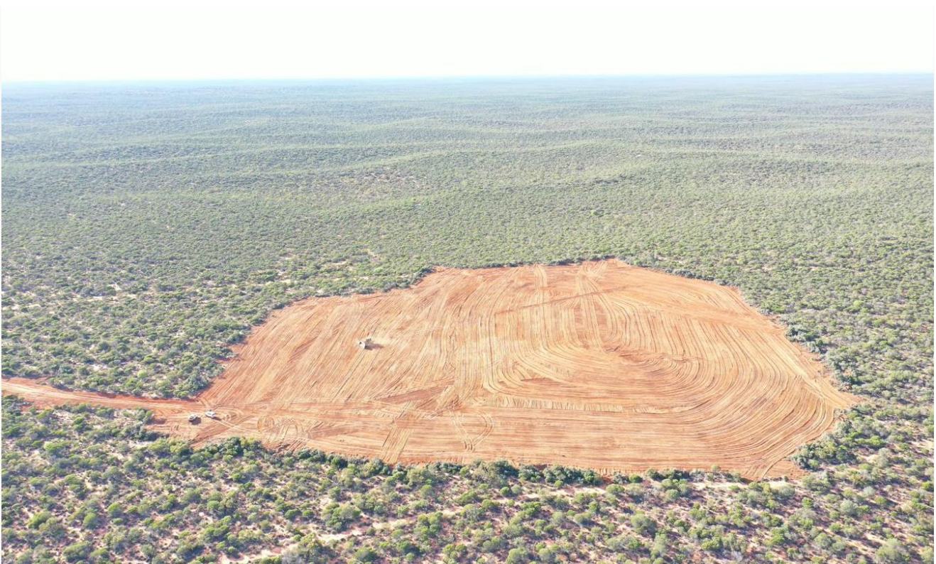
Figure 3 Coburn Project Clearing and Earthworks of the Permanent Accommodation Village Area
