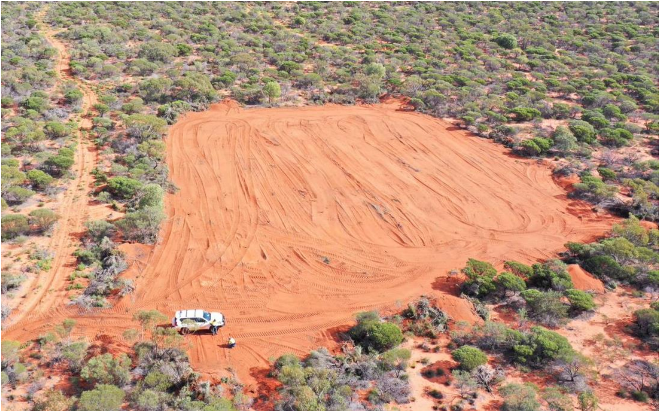
Figure 7 Coburn Project Clearing and Earthworks for the Site Office Administration Area
