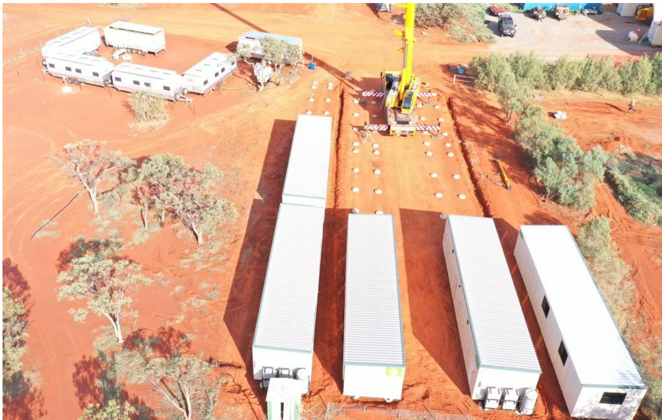
Figure 2 Coburn Project Expansion of Pioneer Camp to support Early Works Construction Activities
