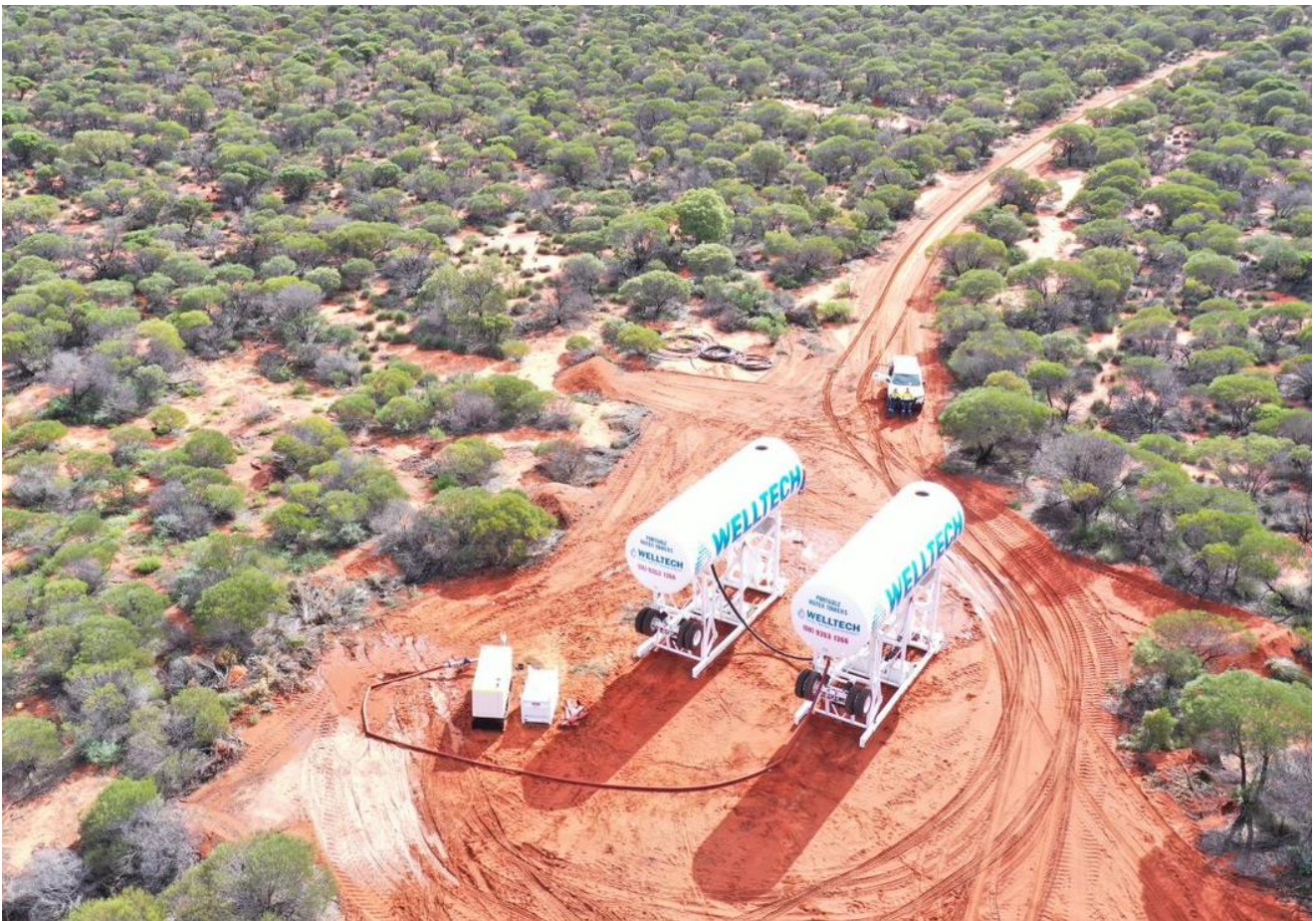
Figure 6 Coburn Project First Production Bore installed, commissioned and ready for use
