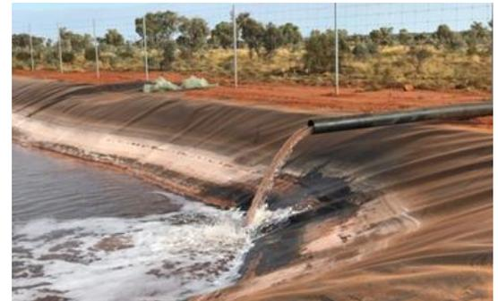
Image: Typical HDPE lined Water Pond
