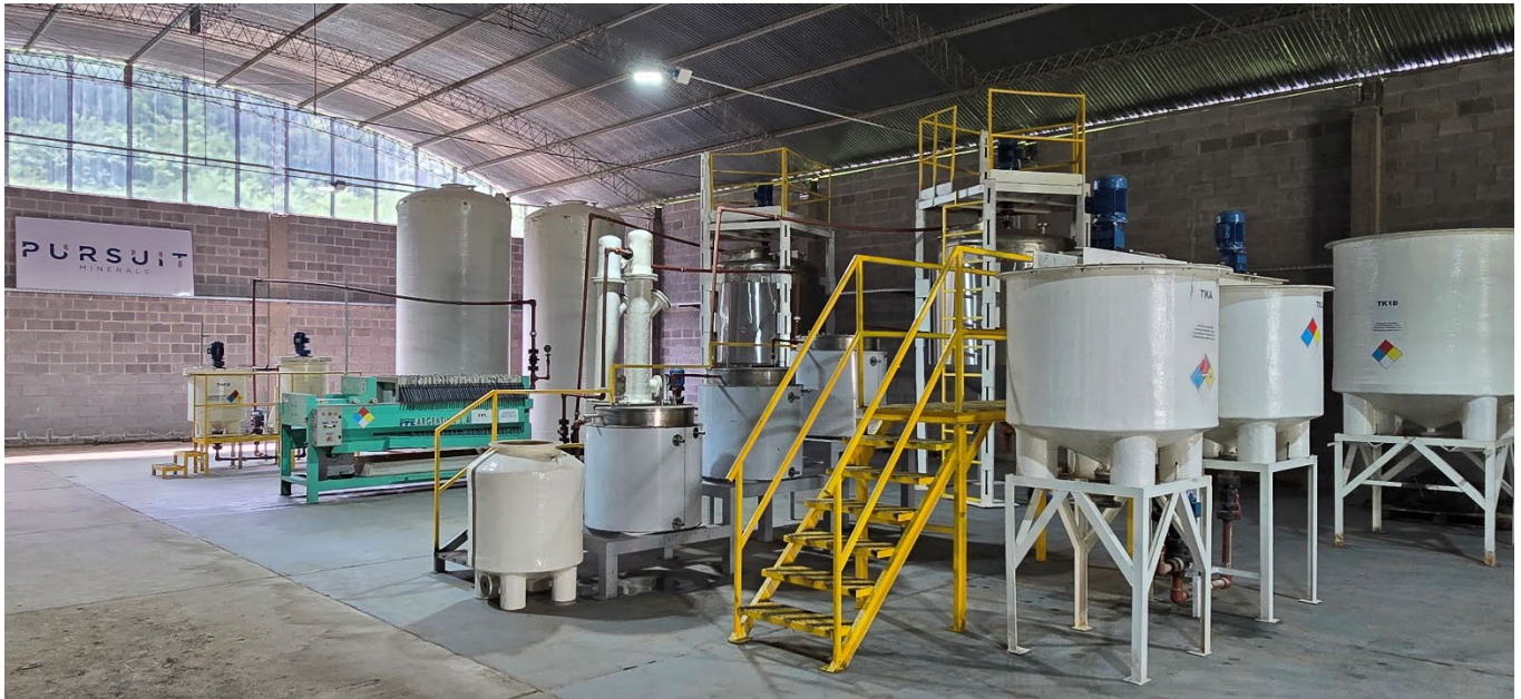
Figure 2 – 250tpa Lithium Carbonate Plant at Pursuit's purpose facility in Salta, Argentina.
