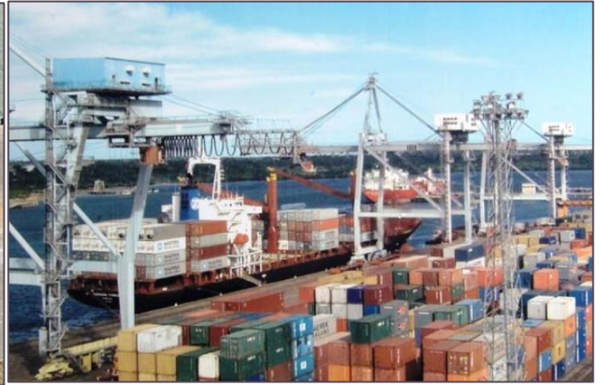
Figure 11: Dar es Salaam Port Container Loading Area
