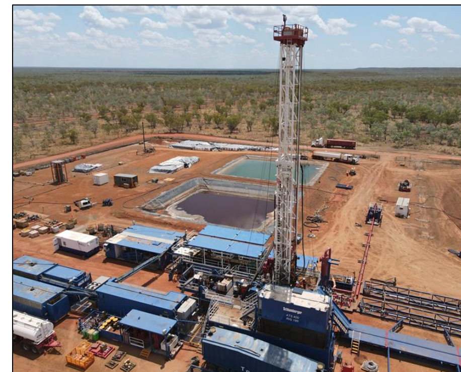
SLB 185 Rig drilling Carpentaria-3H in EP187
