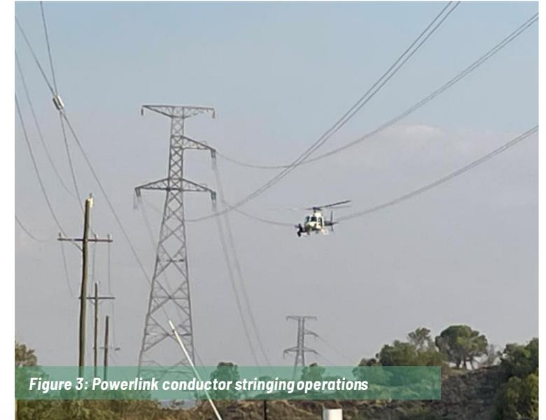
Figure 3: Powerlink conductor stringing operations
