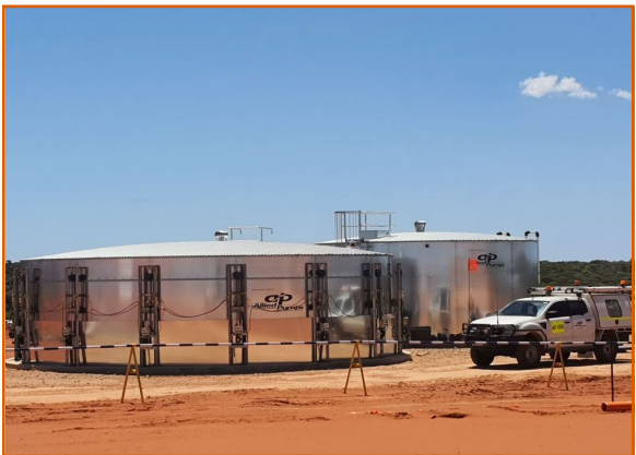
RO Treatment Plant Installation
