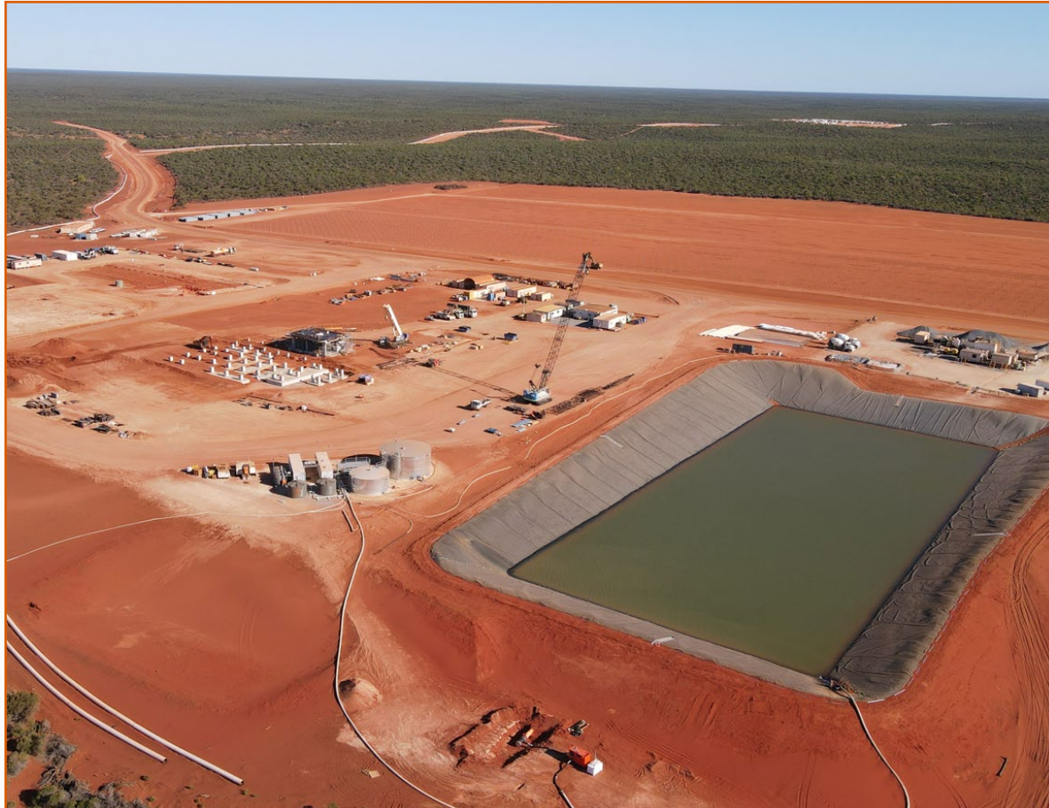
Mineral Separation Plant (MSP) & Hybrid Power Station Area
