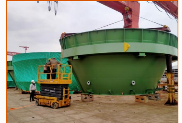
Process Plant Platework Fabrication
