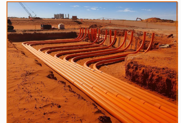
Power Station Conduit Installation
