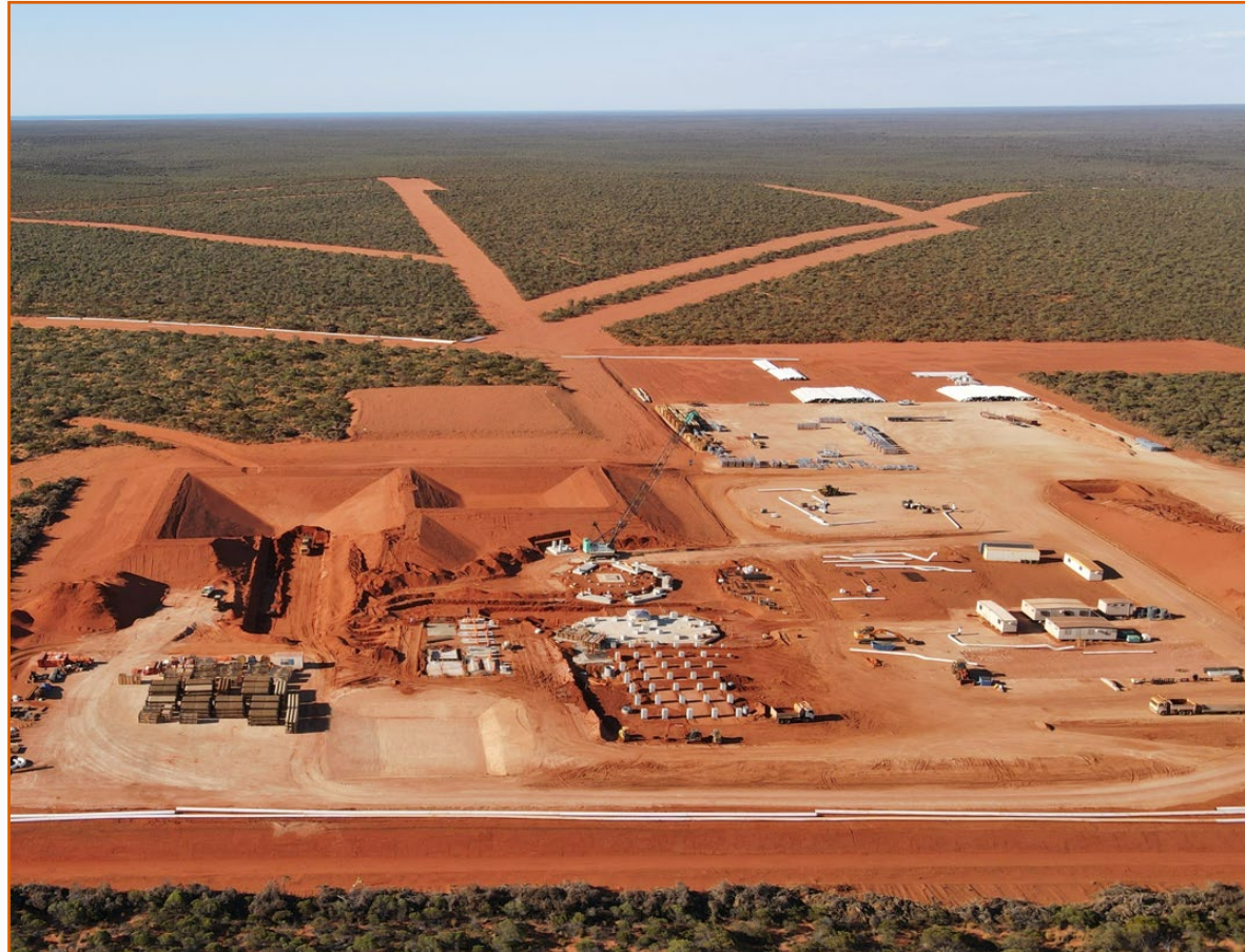
Wet Concentration Plant (WCP) & Mining Area Construction
