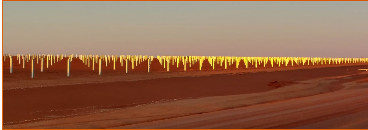
Construction of Coburn's 10MW Solar Farm
