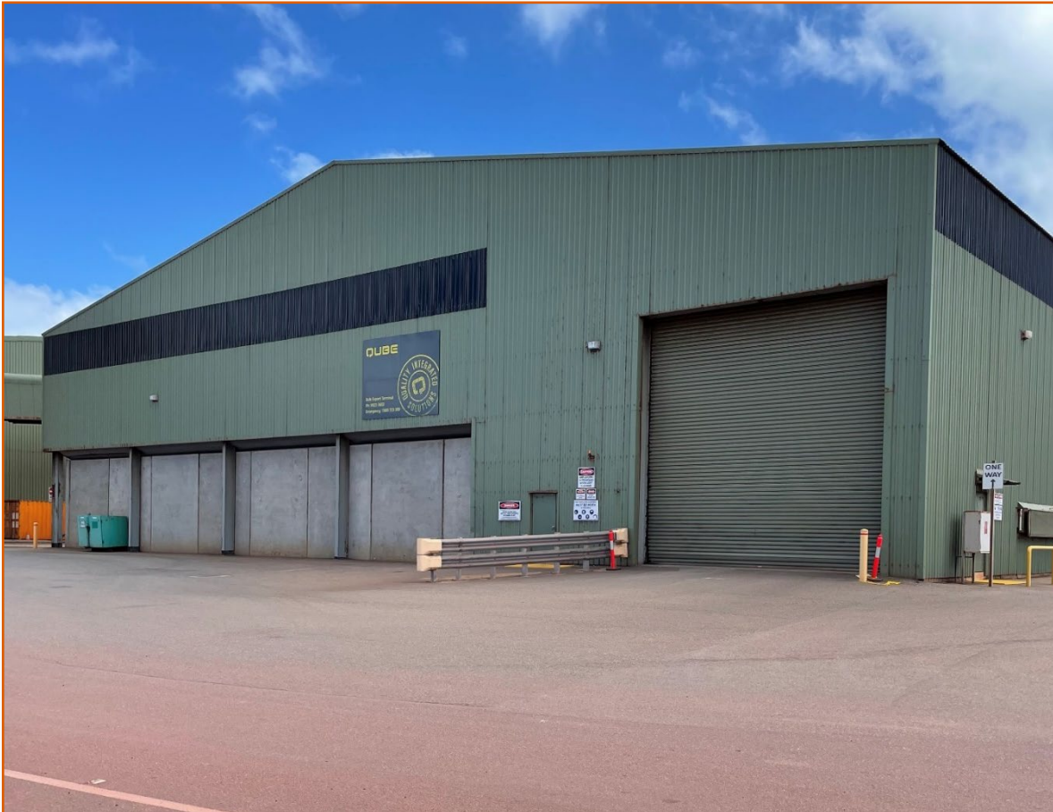
Strandline's Qube Product Storage Facilities at the Port of Geraldton (Berth 4)
