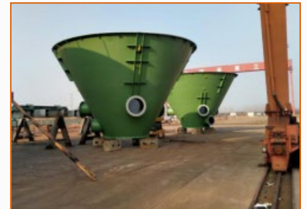
Process Plant Platework Fabrication
