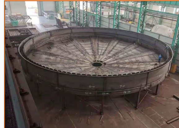
Process Plant Thickener Fabrication
