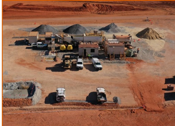
Holcim Concrete Batch Plant Established
