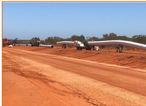
Site-wide HDPE Field Pipe Installation
