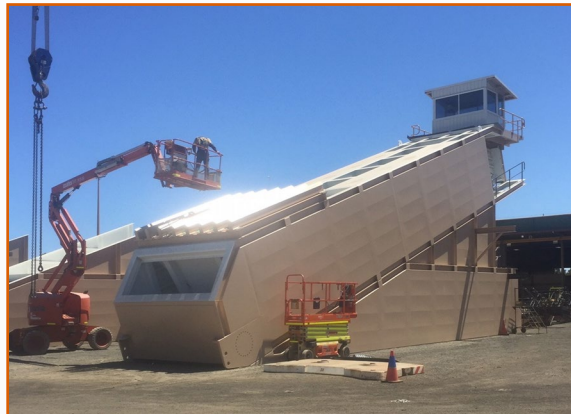
Dozer Mining Unit (DMU) Fabrication
