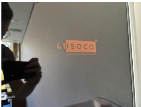
Pattern printed in invisible fluorescent ink in background of clear glass panel.
