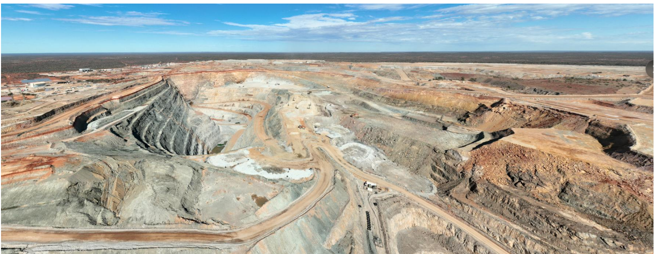
Figure 6: KoTH open pit (looking south west)
