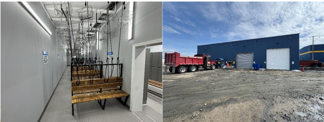
Figure 9: New changeroom facilities and maintenance workshop
