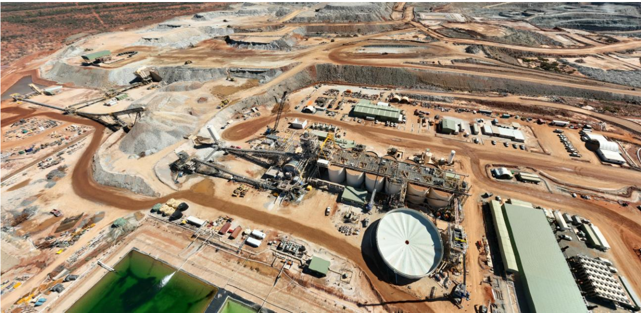
Figure 7: KoTH stage 1 plant upgrade project – New crusher installation (LHS) and 4* additional tanks added to the wet plant (RHS)
