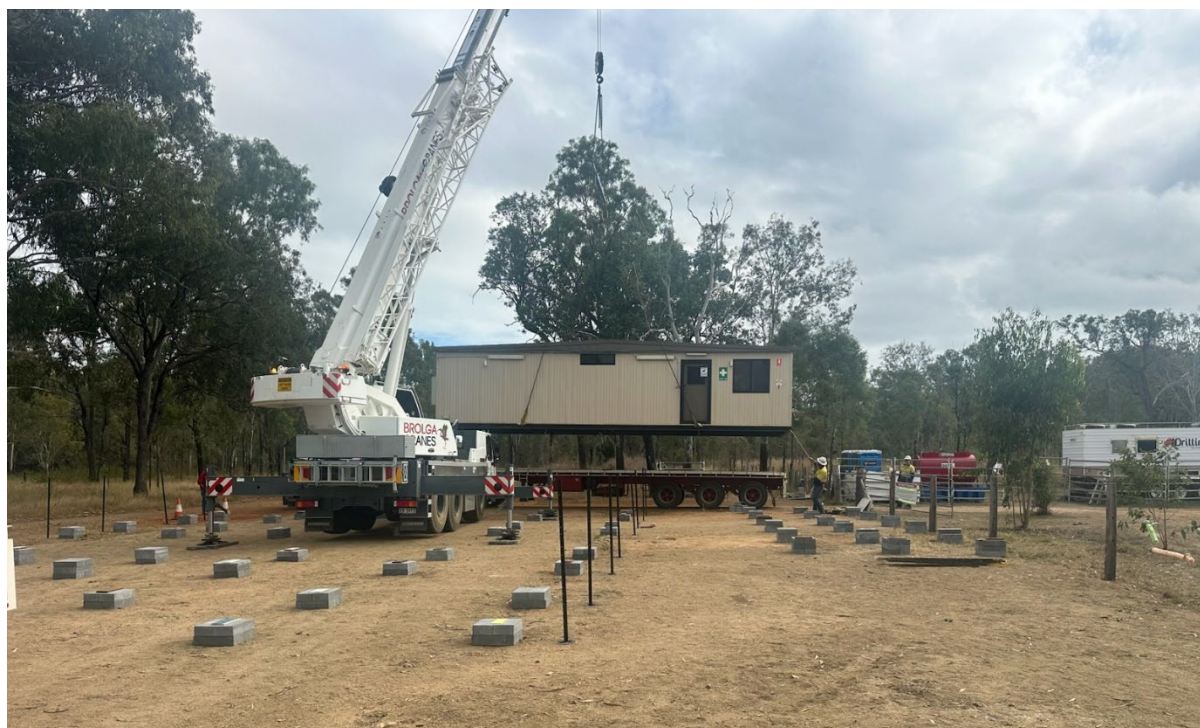
Figure 1 Kitchen/Messing Block being moved into position at Briggs.
