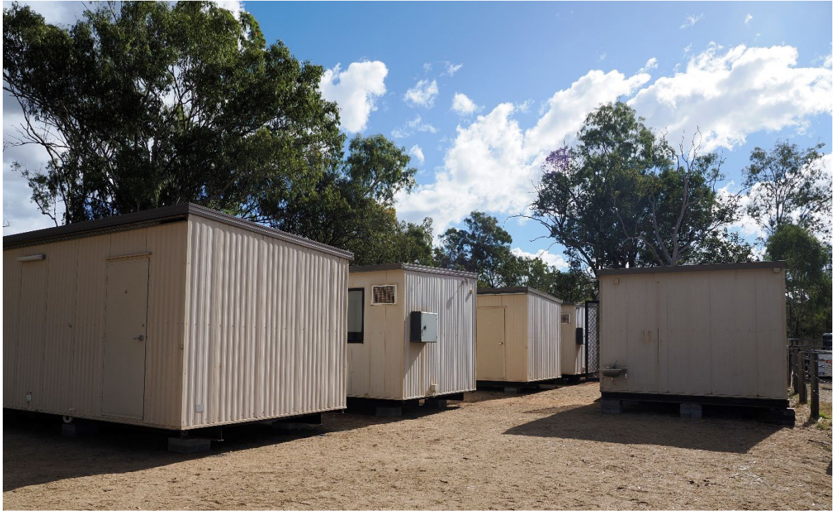
Figure 2. Four accommodation blocks in place next to kitchen/messing block. Covered walkways to be installed during commissioning.
