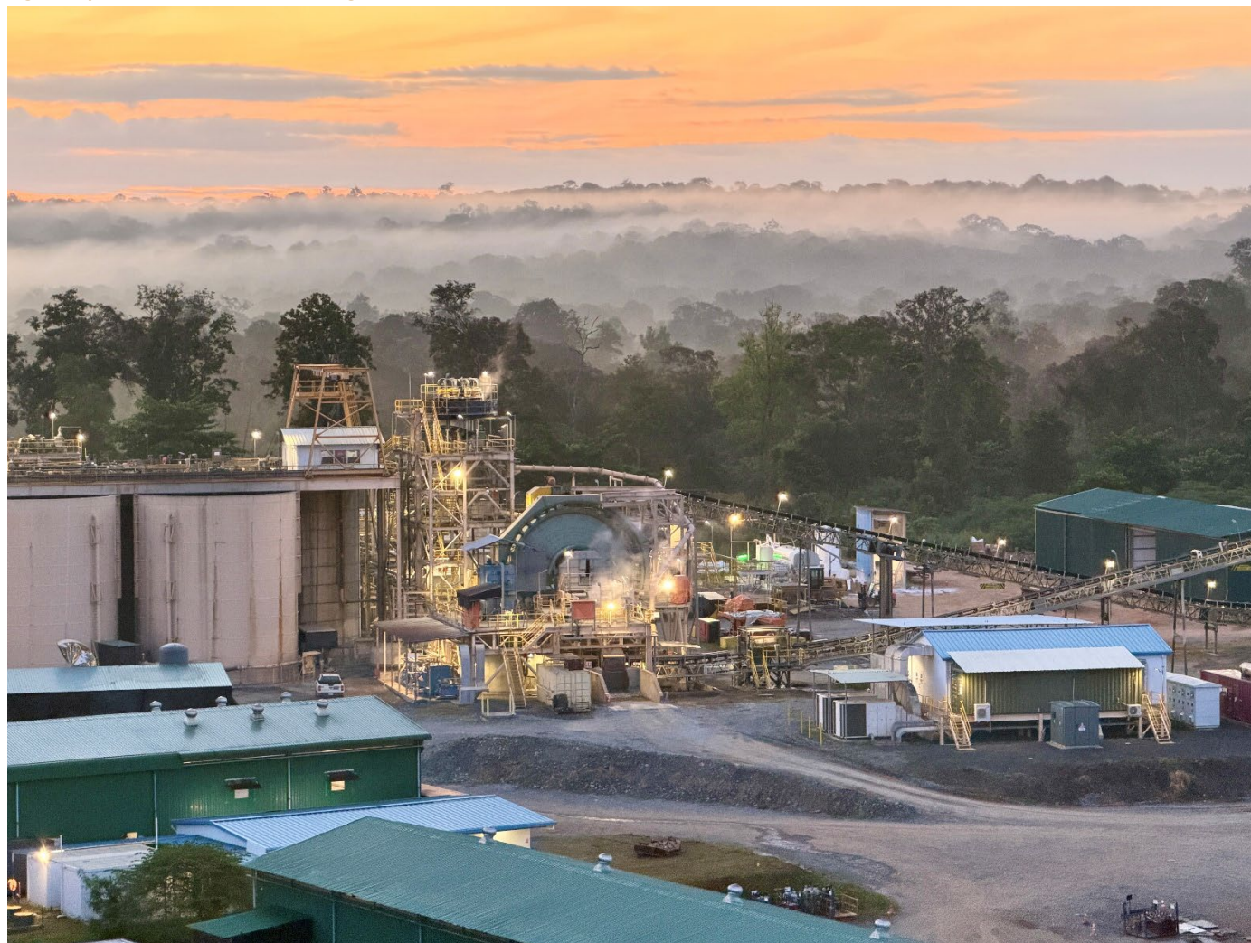
Figure 1 | Okvau Gold Mine Processing Plant
