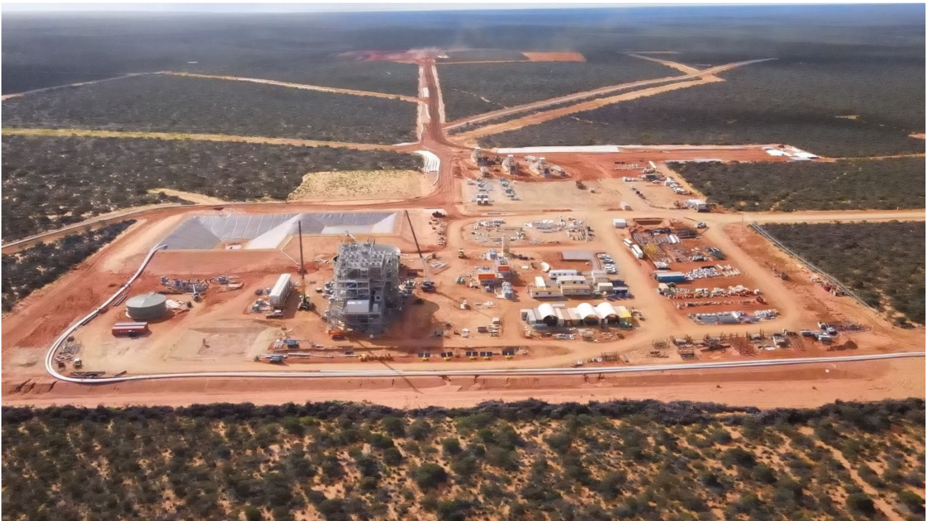
Figure 1 Construction of Strandline's 100%-owned Coburn mineral sands project is progressing rapidly
