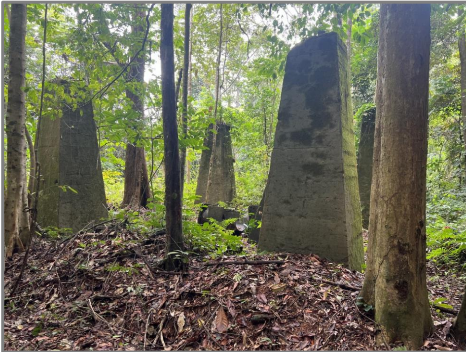
Crusher footings discovered in 2022 reconnaissance mapping
