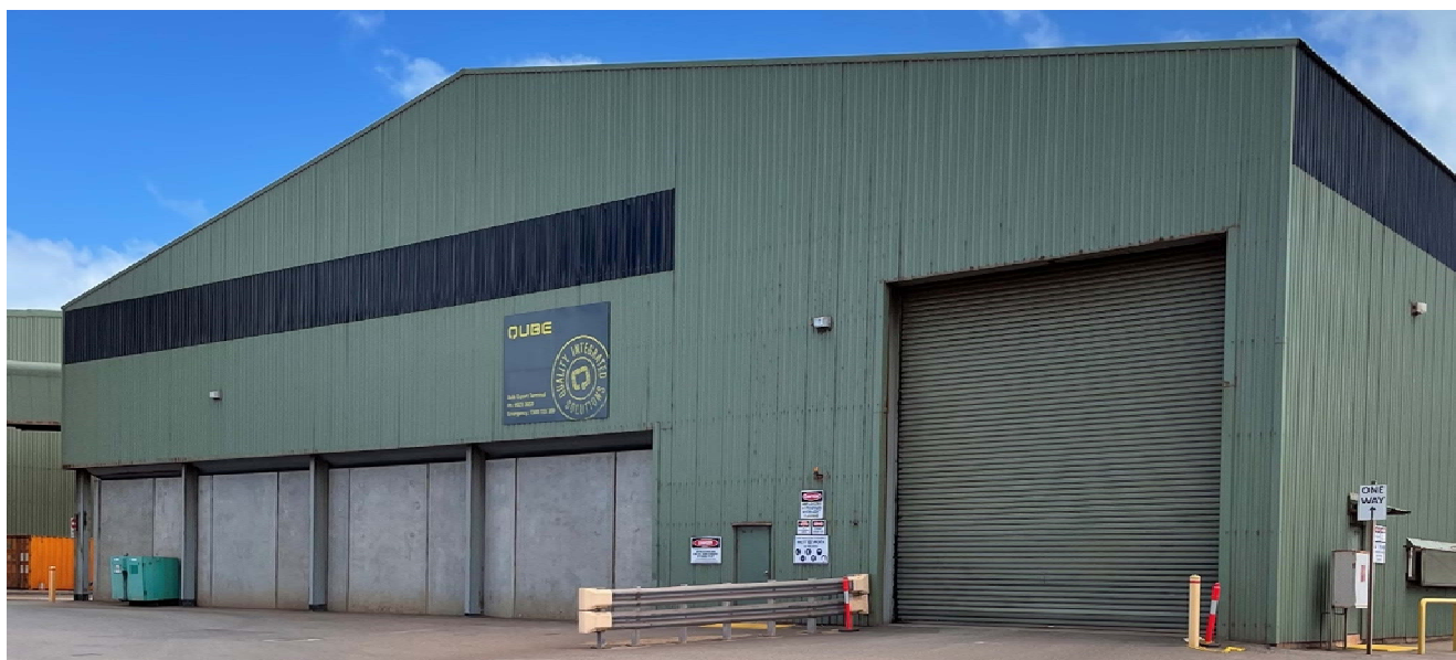
Figure 2 Strandline’s Qube product storage facilities at the Port of Geraldton (Berth 4)
