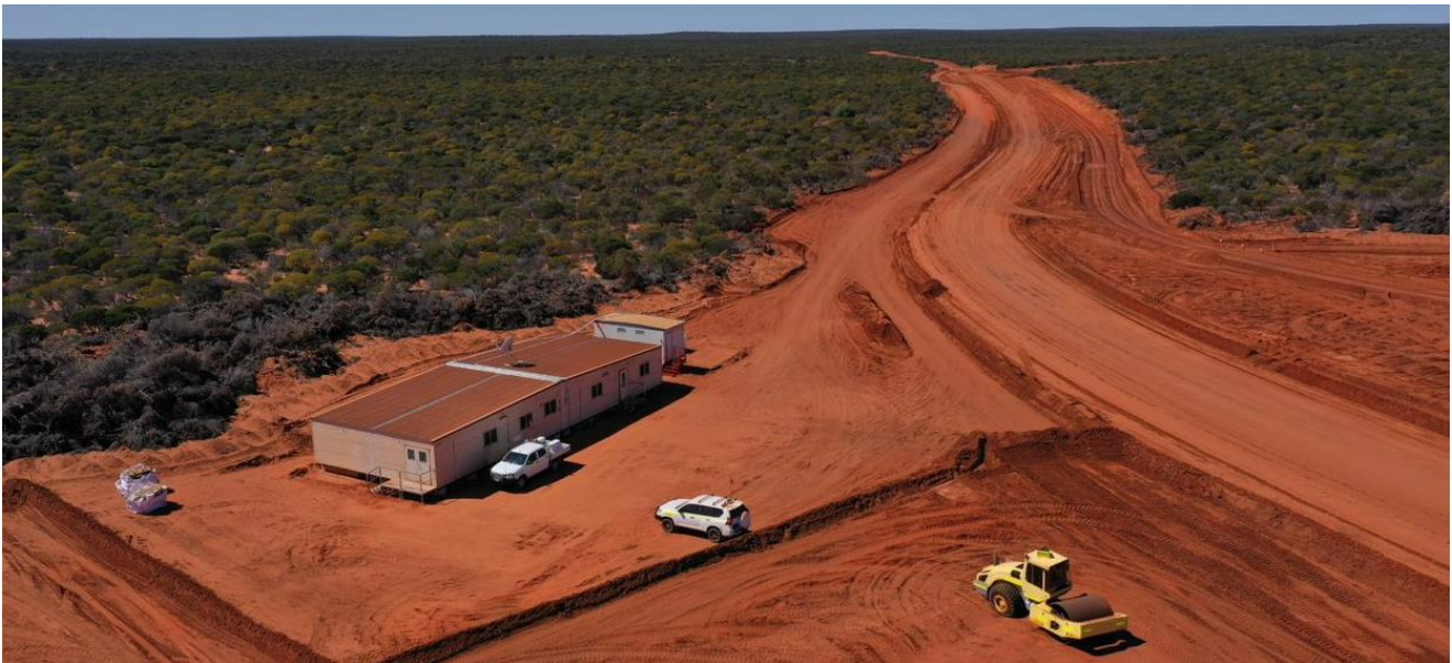
Figure 11 Strandline's Construction Office Commissioned at the MSP Area
