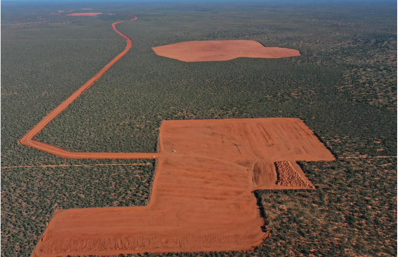
Figure 3 Wet Concentration Plant (WCP) Bulk Earthworks Pad
