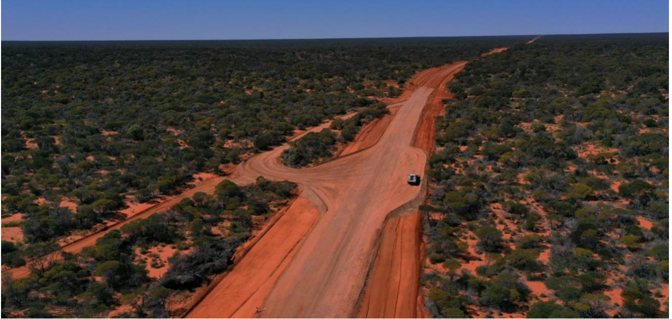
Figure 8 Main Access Road Construction Continuing with Installation of Road Base Material
