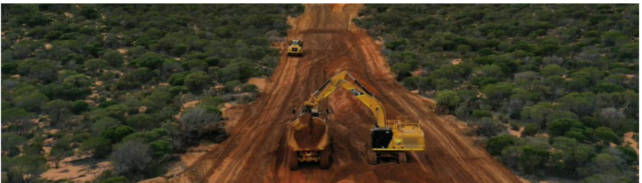
Figure 10 Main Access Road Construction Continuing
