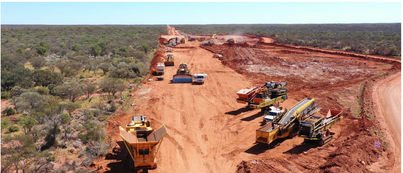
Figure 7 Borrow Pit Established and Production of Base-Course Material Underway
