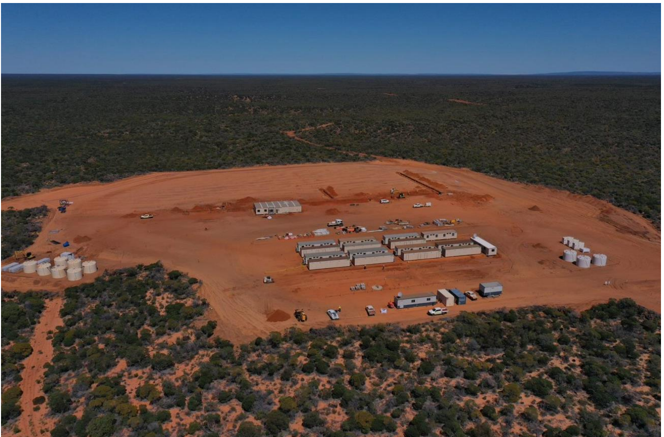
Figure 4 Construction of x270 person Accommodation Village Advancing Rapidly
