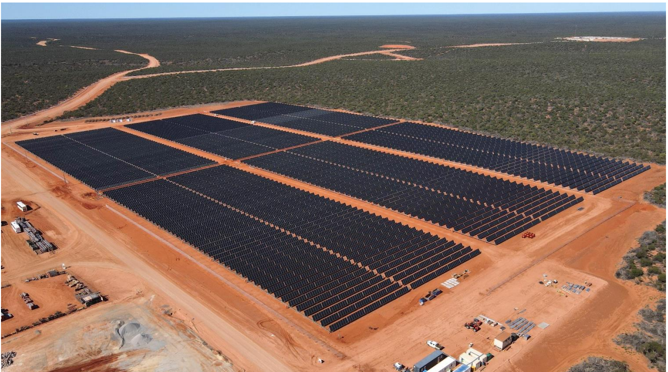
Figure 4 Coburn Project 11MW Solar Farm installed by Pacific Energy
