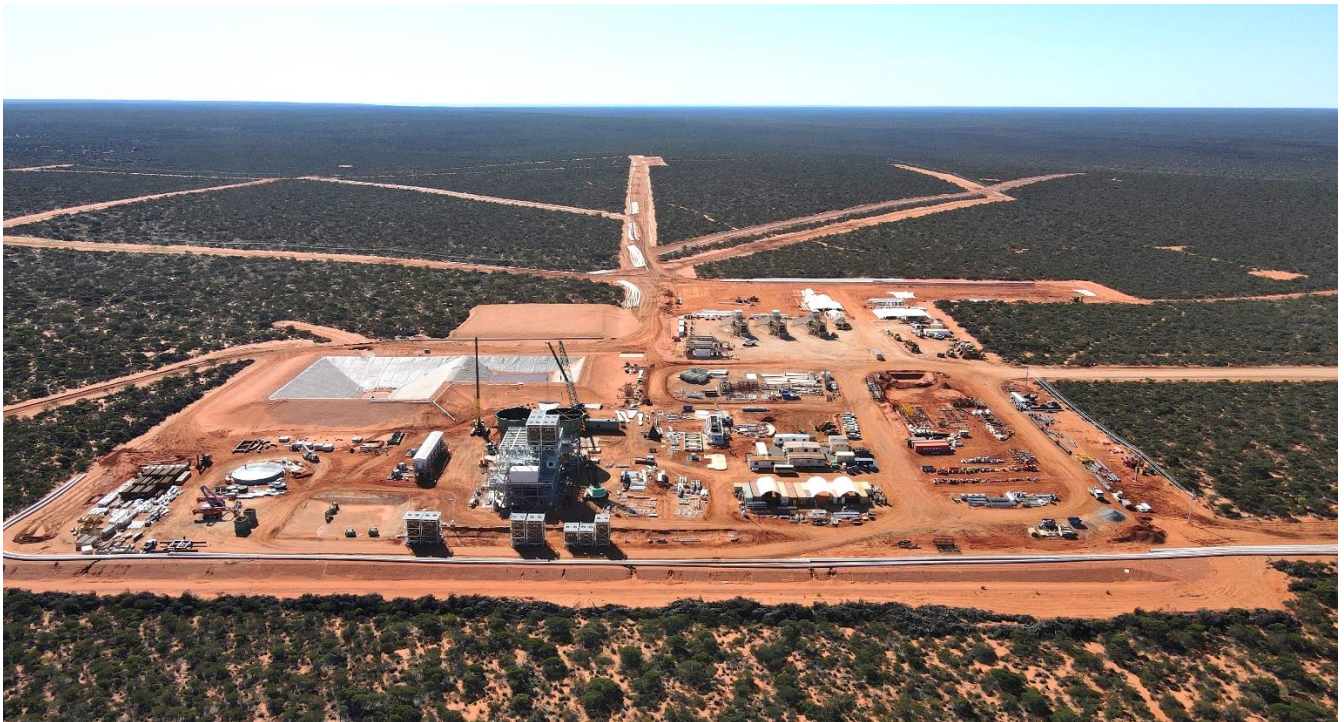
Figure 1 Coburn Project Wet Concentration Plant Area Progress Photos
