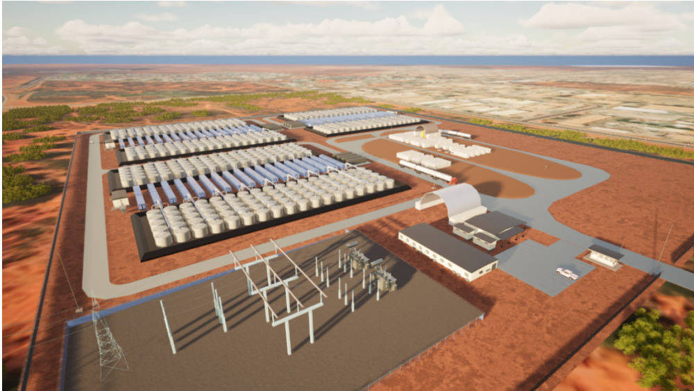
Figure 1: Conceptual render of a potential 50MW / 10-hour (500MWh) vanadium flow battery configuration for the Kalgoorlie VBESS project
