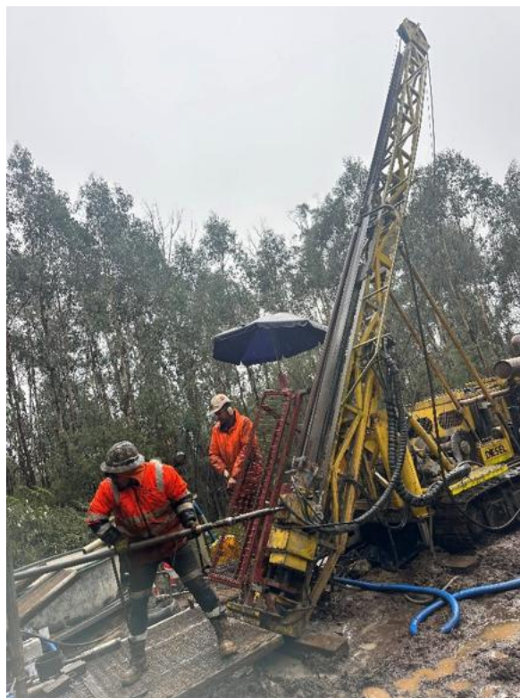
Figure 2: Drilling underway of 26SSDH004
