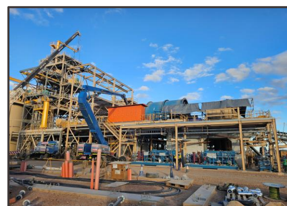
Ball mill installation
