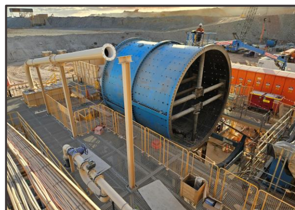
Ball mill installation
