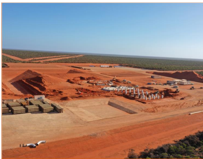
Wet Concentration Plant (WCP) Concrete Foundations Progressing
