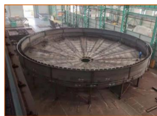
Process Plant Thickener Fabrication
