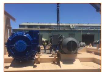
DMU Pump Skid Fabrication
