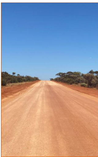
42km Main Access Road Construction
