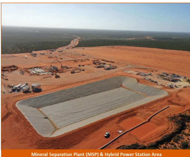
Mineral Separation Plant (MSP) & Hybrid Power Station Area
