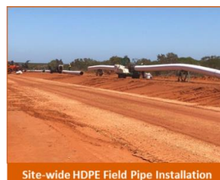
Site-wide HDPE Field Pipe Installation
