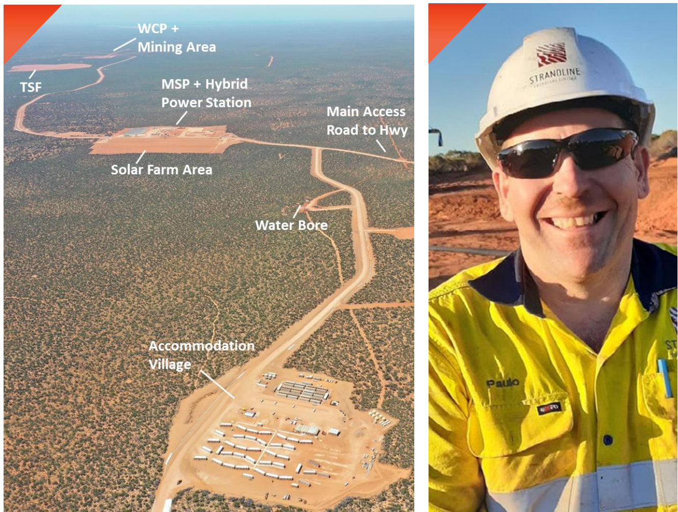
Figure 2 Coburn site wide construction progressing strongly (Jan-2022)
