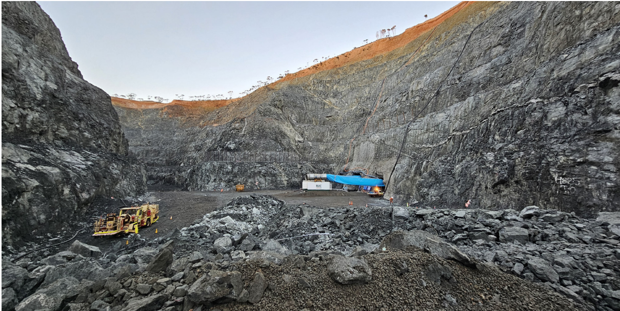
Picture – Scotia Operations showing portal in background.
