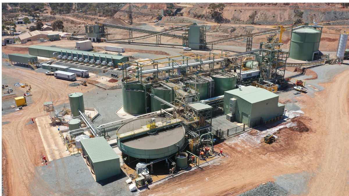
Picture – Norseman Processing Facility.
