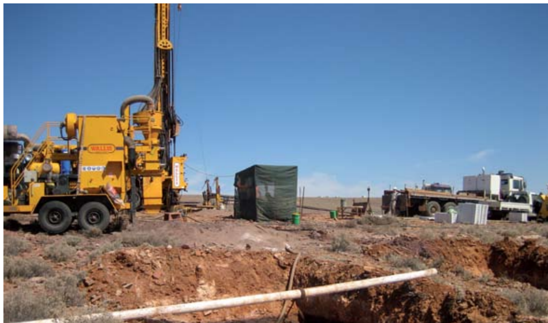
Drilling of MGD 49 at Mount Gunson, March 2009
