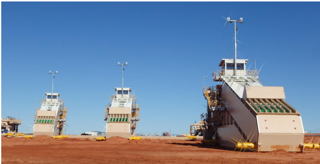
Figure 1 Three (3) In-pit Dozer Mining Unit Supplied & Assembled on Site by Piacentini&Sons
