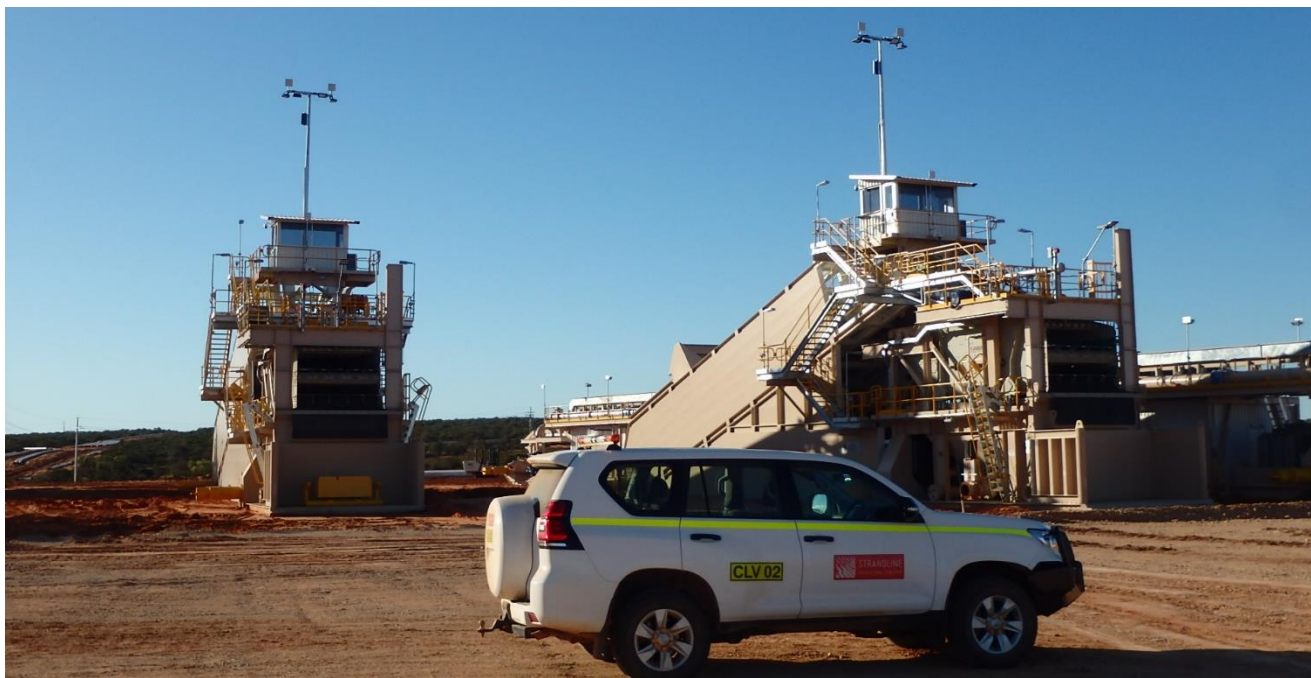
Figure 2 Dozer Mining Units prepare the ore for slurry pumping to the WCP. Sand tails from the WCP is returned to the pit void, contoured and rehabilitated
