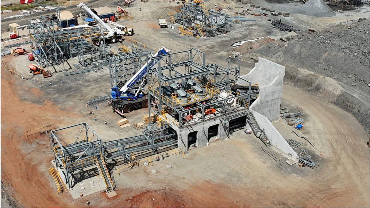
Photo 3: Primary crusher area concrete and structural steel, with major equipment installed.
