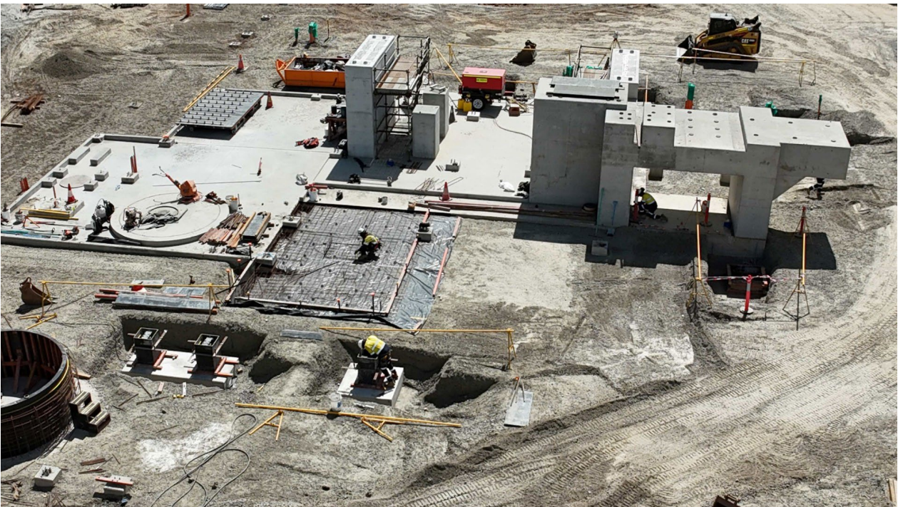
Photo 4: Ball mill area major concrete complete.
