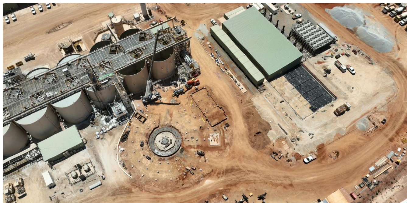
Wet plant & power station
