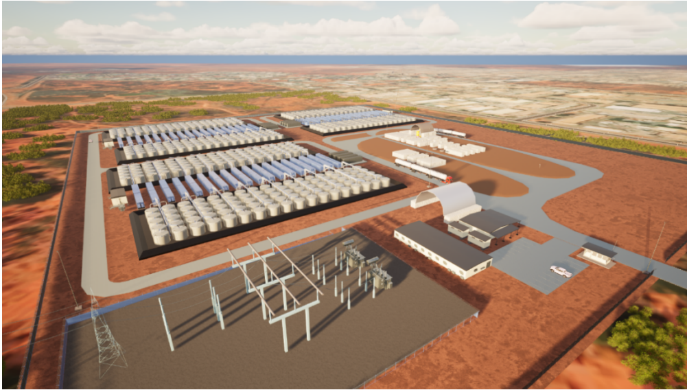
Figure 1: Render of a 50MW-10h (500MWh) vanadium flow battery for the Kalgoorlie VBESS project
