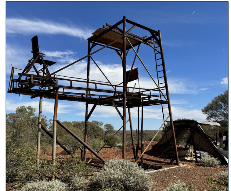
Barrambie Range North Shaft c.1970's
