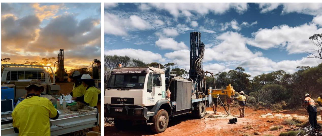
Figure 3 – Aircore drilling at the T8 prospect
