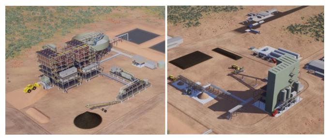
Figure 1 Coburn Preliminary 3-D Engineering Model of Wet Concentration Plant (WCP) and Mineral Separation Plan (MSP) Infrastructure
