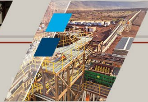
LOAD OUT INFRASTRUCTURE
