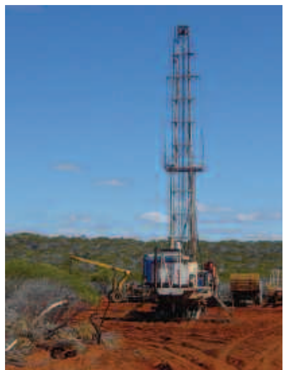
Water rig drilling hole CPB3 at Coburn. For location, see Figure 5.
