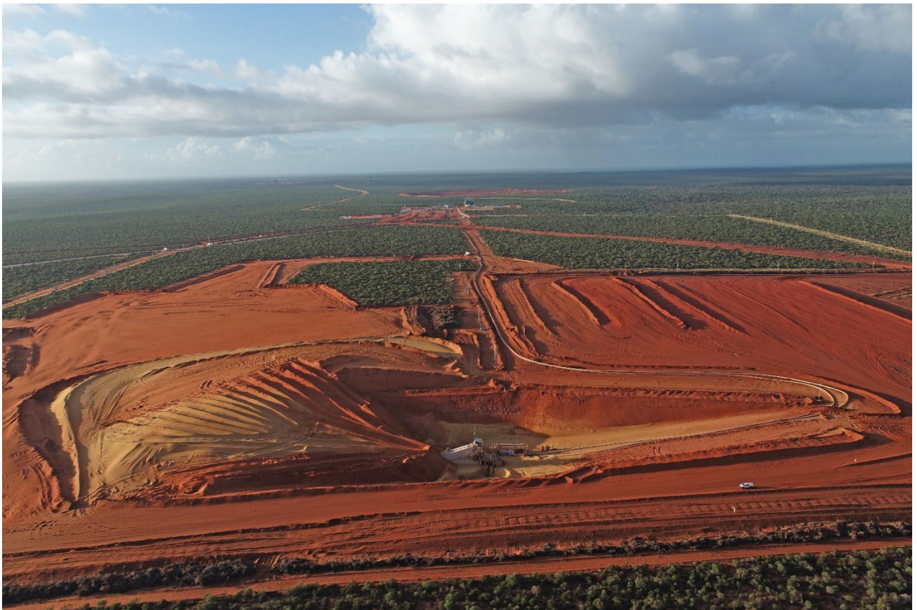
Figure 5 Coburn Open Pit Mining of Ore has Commenced. Ore is Pumped in Slurry Form approximately 1-2km to the WCP
