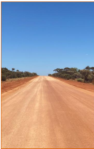
42km Main Access Road Construction
