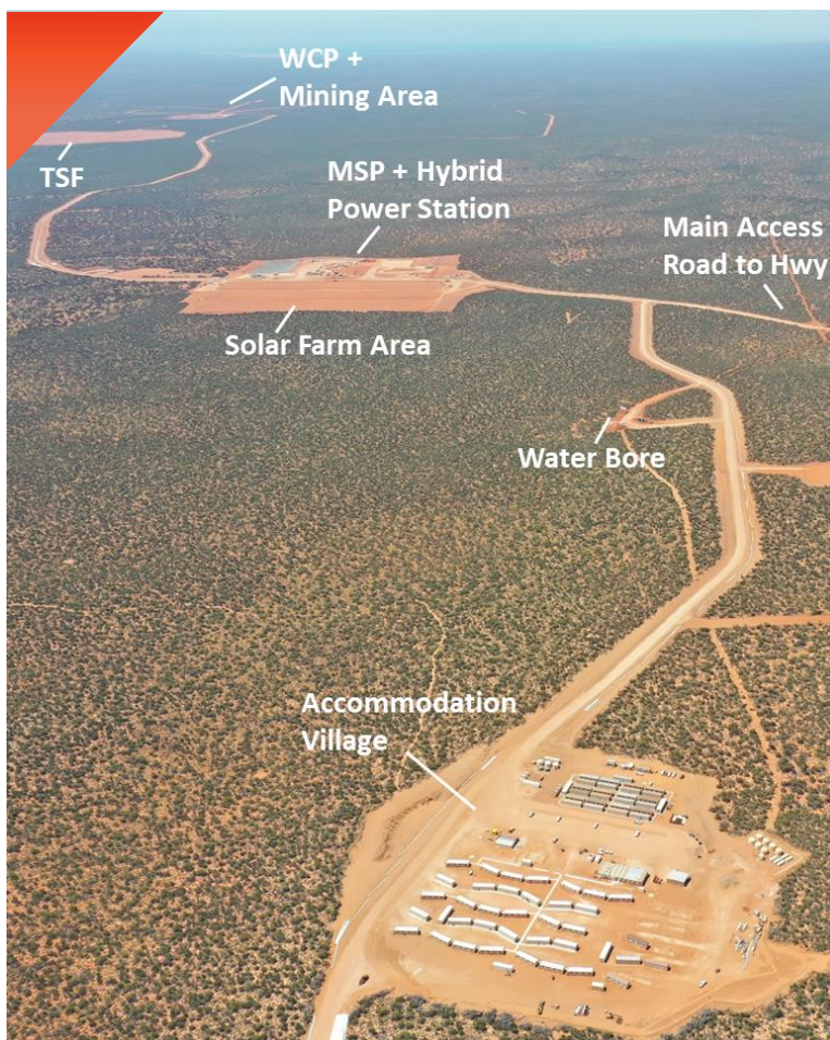
Figure 3 Coburn site wide construction progressing strongly (Jan-2022)
