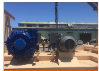
DMU Pump Skid Fabrication
