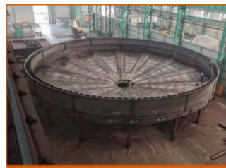
Process Plant Thickener Fabrication
