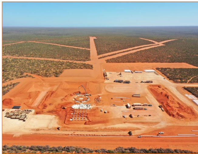
Wet Concentration Plant (WCP) Concrete Foundations Progressing
