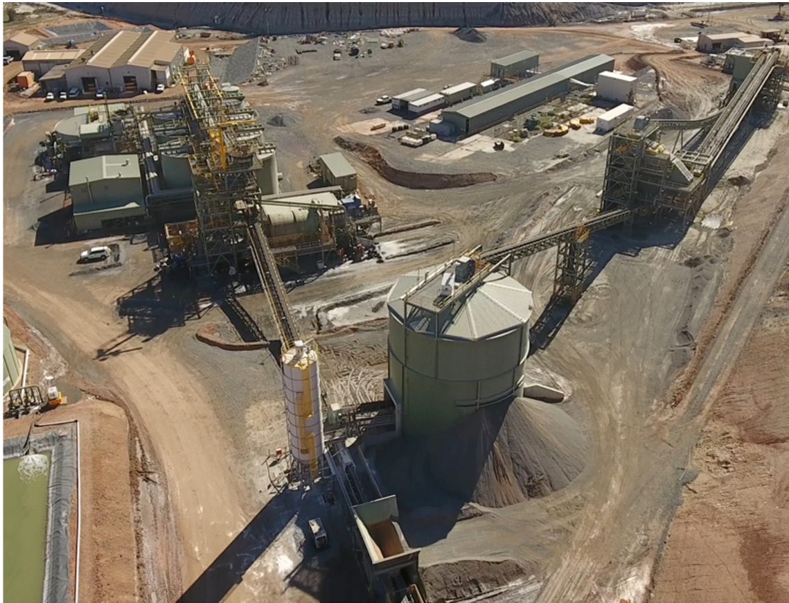
Norseman processing plant currently operating at 1.2Mt per annum
