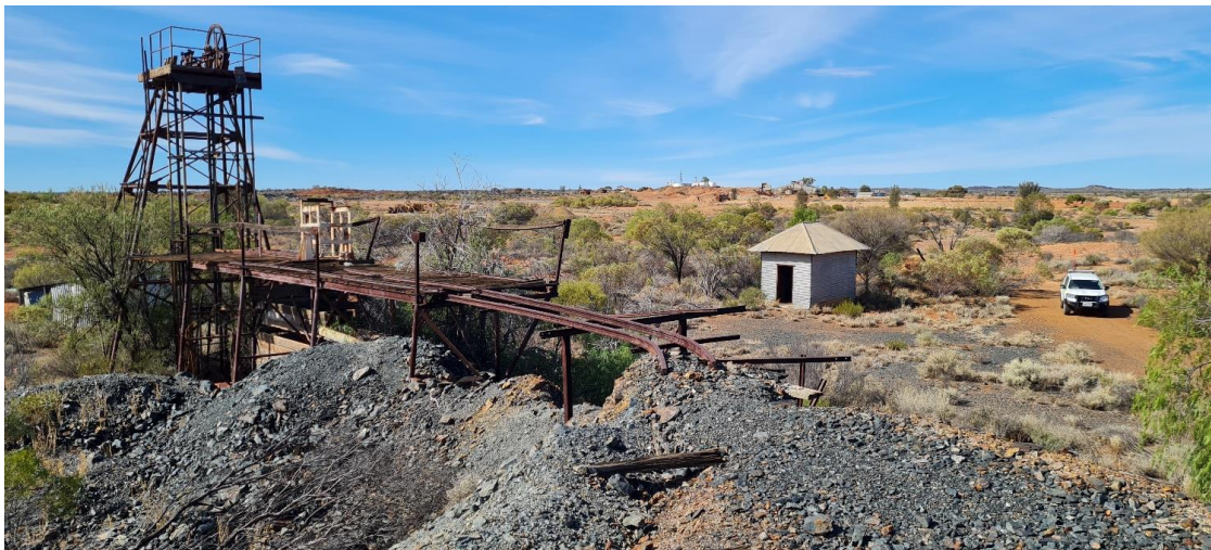
Figure 6 - Aspacia Headframe (looking South East)
