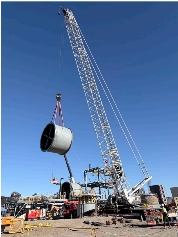
Photos 1 and 2. Installation of the new ball mill at Eloise copper mine.
