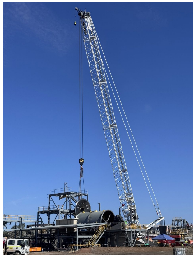
Photos 1 and 2. Installation of the new ball mill at Eloise copper mine.
