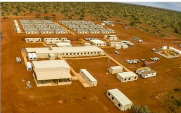
Image: Typical Site Accommodation Village
