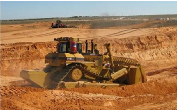
Image: Typical dozer push operation
