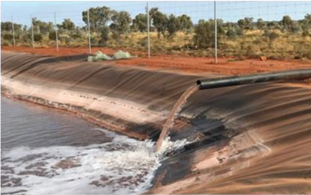
Image: Typical HDPE lined Water Pond
