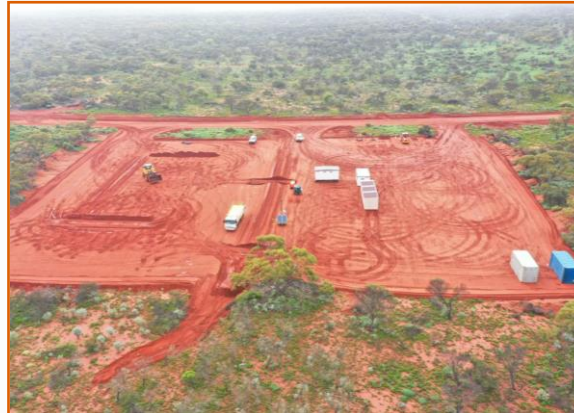
Preparing Construction Laydown Area
