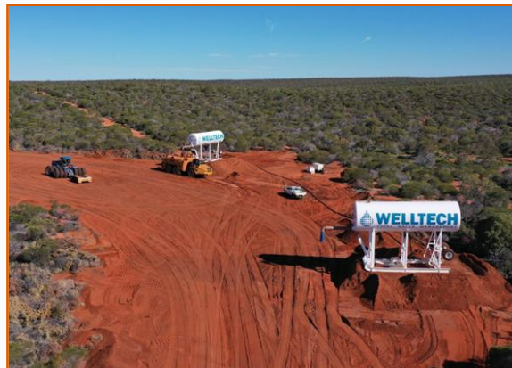
First Production Bores
