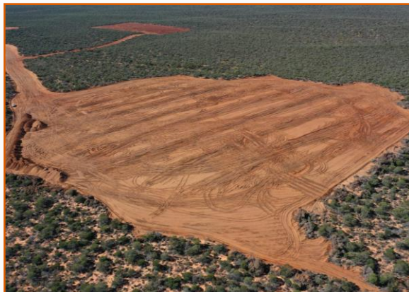
Village Bulk Earthworks Pad
