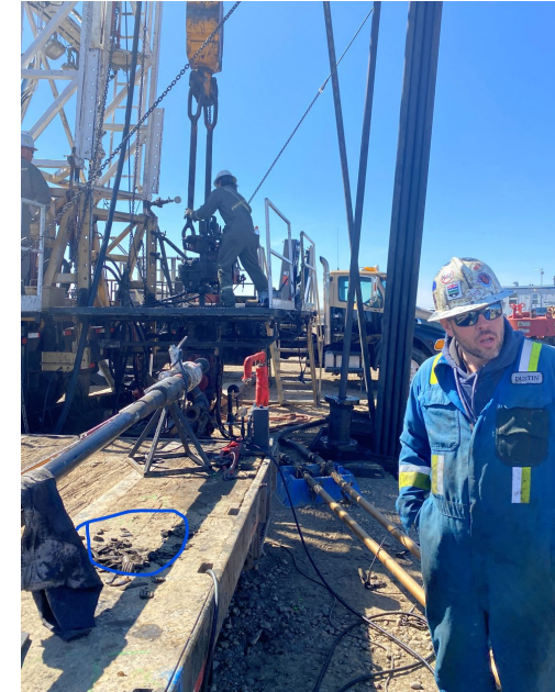
Workover completed at 2-29 to increase water disposal capacity to >12,000 bbl/d
