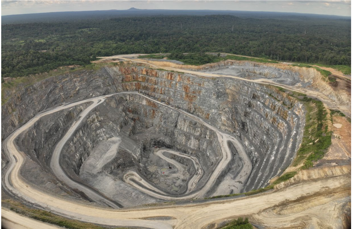
Figure 1 | Okvau Open Pit – October 2025
