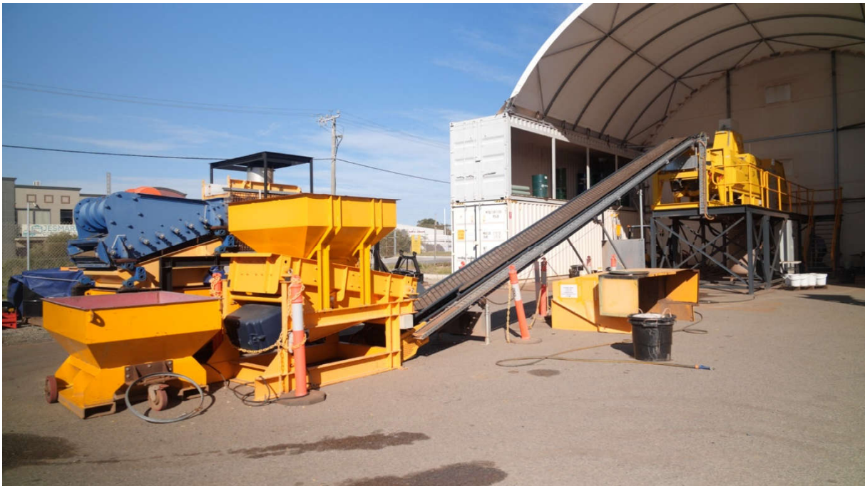
Figure 1: Ore sorting facility used during testwork is the same size proposed for use at Kayelekera
