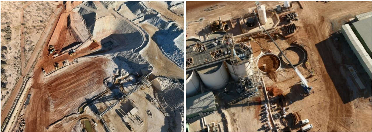
Figure 6: Stage 1 upgrade works underway with crusher excavation work (left) and new tank footings (right)
