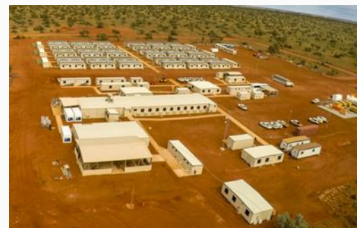
Image: Typical Site Accommodation Village
