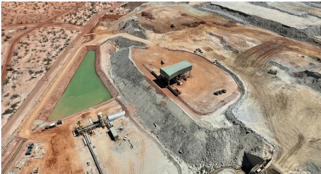
Figure 1: New crusher installation
