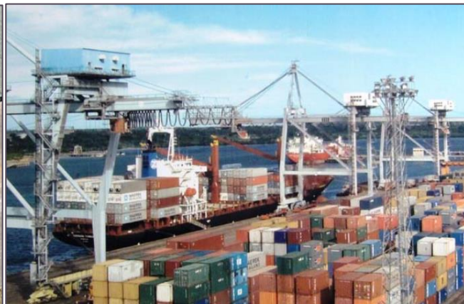
Figure 11: Dar es Salaam Port Container Loading Area
