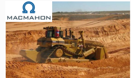
Image: Conventional dozer push mining operation
