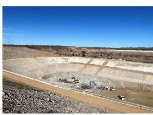
Figure 6: Preparatory Works for the Intake Shafts
