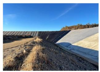
Figure 5: Wises Dam Liner Installation
